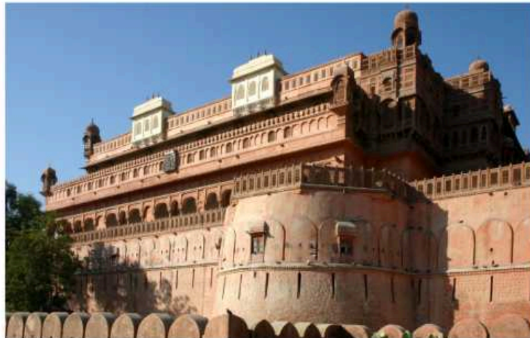
Junagarh fort at Bikaner (source: Wikipedia)
