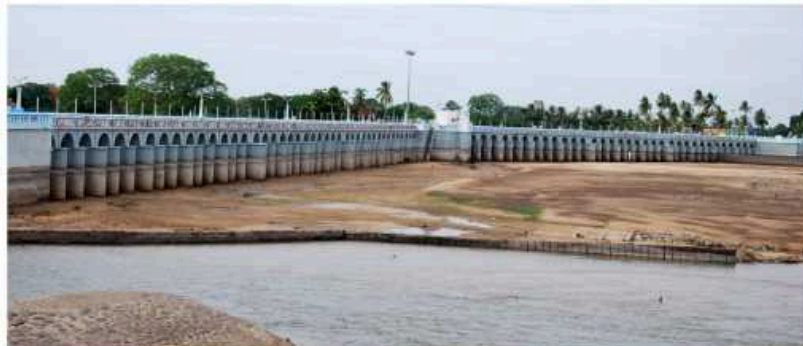
The 329-metre-long 'Grand Anicut' ( Kallanai in Tamil) across the Kāveri River, thought to have been constructed by the Chola king Karikāla some 1,800 years ago (it has been restored several times since), is a massive and effective water-diverting device, splitting the river into four streams and irrigating thousands of hectares of agricultural land in the Kāveri delta. (Courtesy: Michel Danino)
